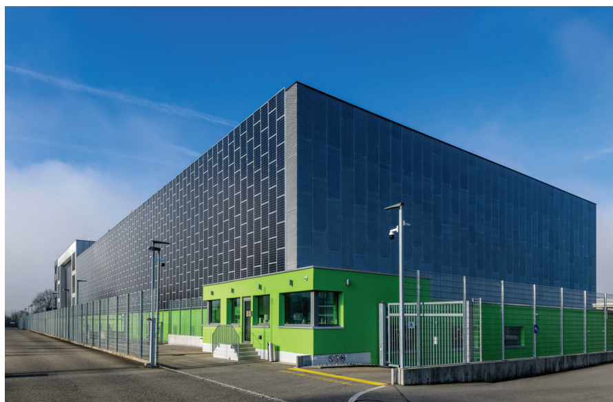
Green has launched its own green initiative, whereby it feeds the waste heat from the data centre into a specially designed heating network to be used for public heating purposes.
